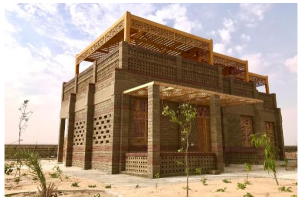
- Affordable housing unit built in 2024 at Al-Kharga city, The New Valley Governorate, designed by Dr. Nermine Abdel Gelil.
