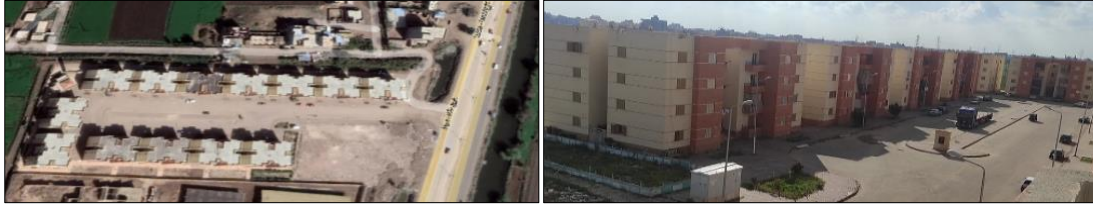
(A)- The Outskirts Social Housing Project in Kafr Saad City (400 Units). Source: Google
